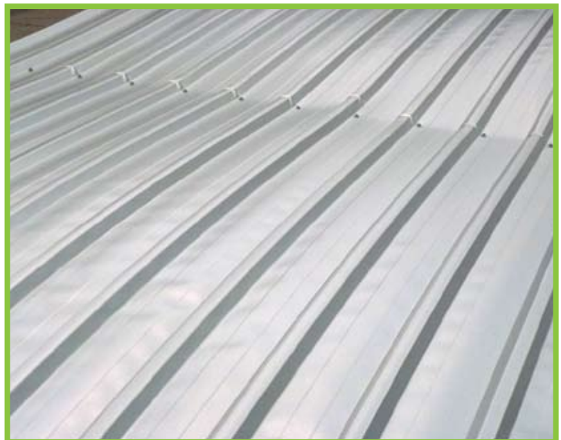
Wall Pressure Test
